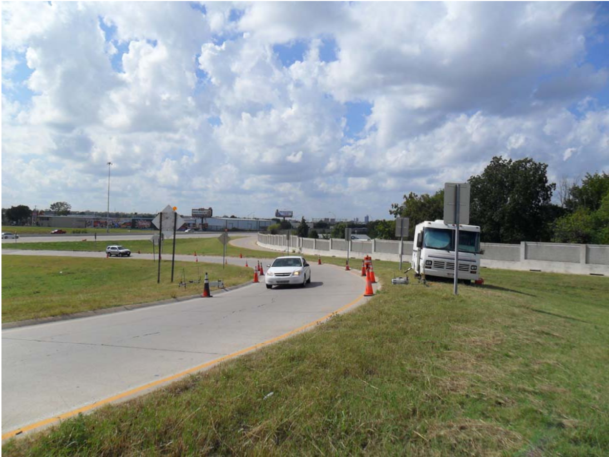
Figure 2. Tulsa 2013 monitoring site looking west toward downtown Tulsa.
